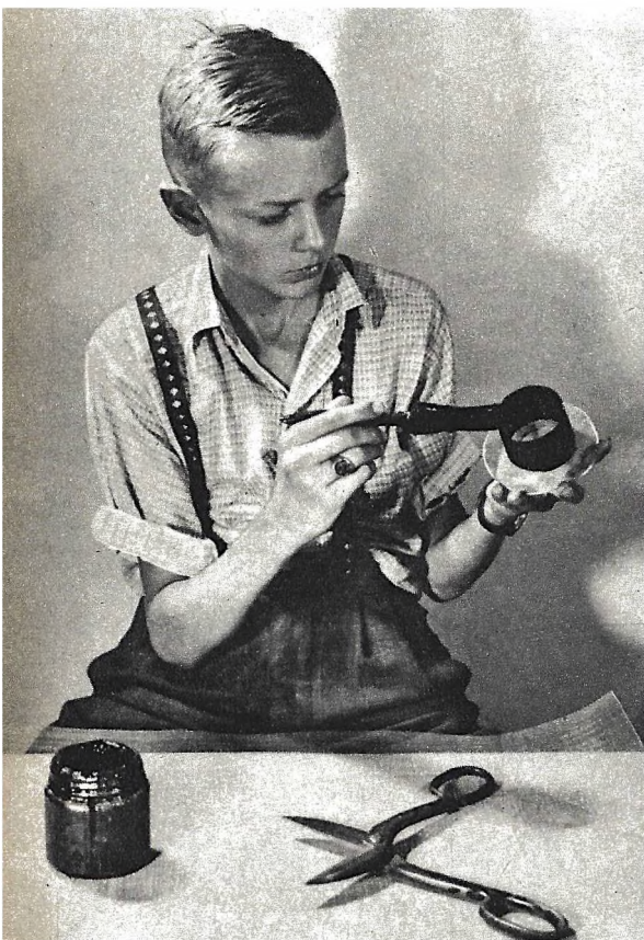
Coating the sides of a neat, practical ash receiver with asphalt varnish. Baking it will give a very hard and lustrous finish particularly suited to ash tray use.
